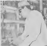
Jacinto Croeze wears asbestos gloves to pull out a burner gun from boiler at the Edeleanu Plant. Jacinto Croeze ta bisti handschoennan di asbestos pa saca "burner gun" for di un boiler na Edeleanu Plant.
